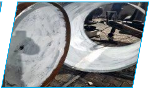
Epoxy Coating Inside Tanks
