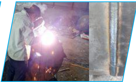
Welding Process by Skilled Operator
